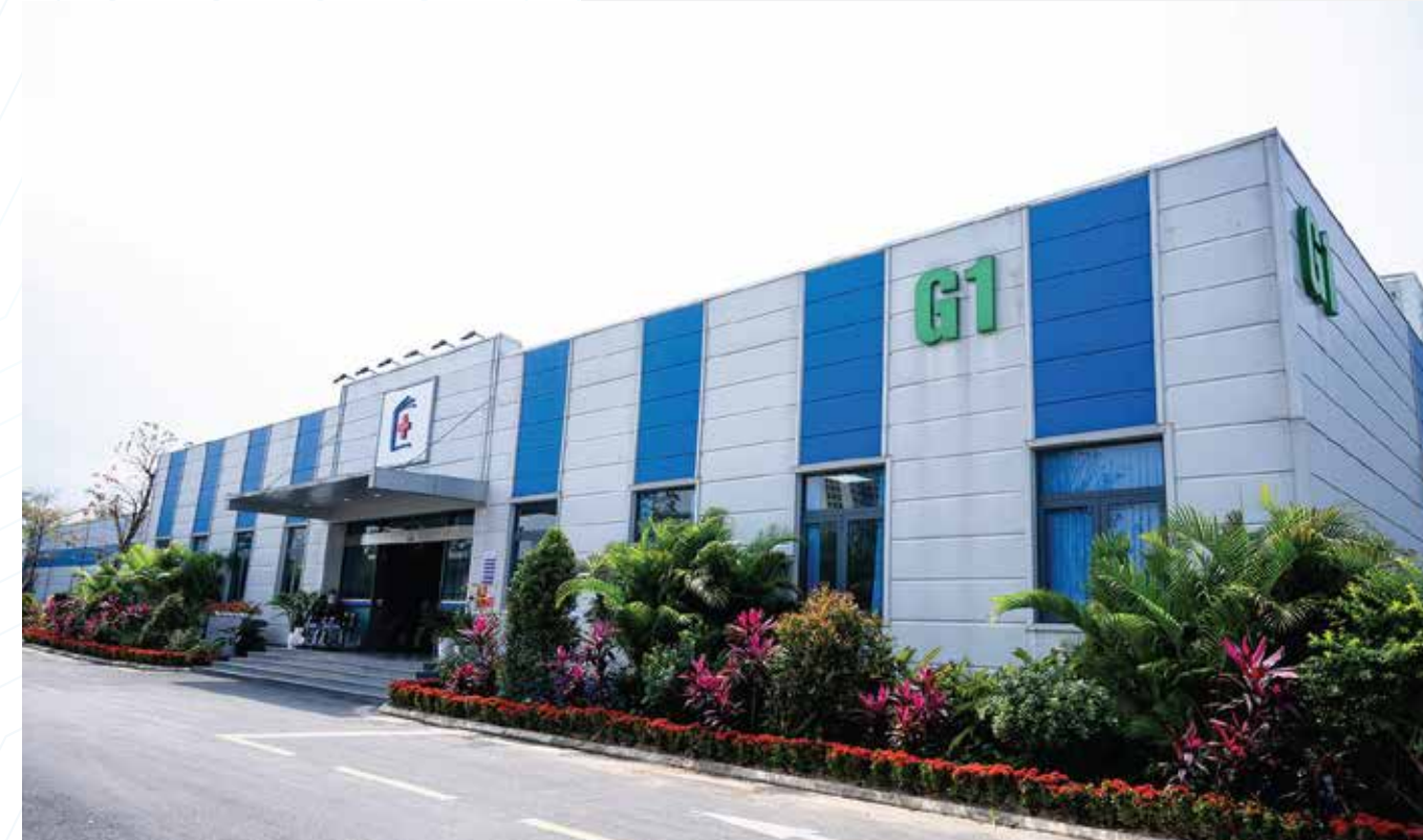
Covid-19 hospital treating severe and critical patients Completion after 30 days
